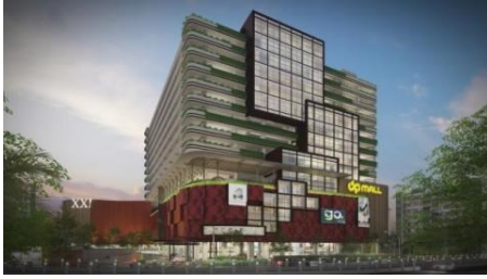
Gambar 1. Tampilan Gedung DP Mall Expansion
