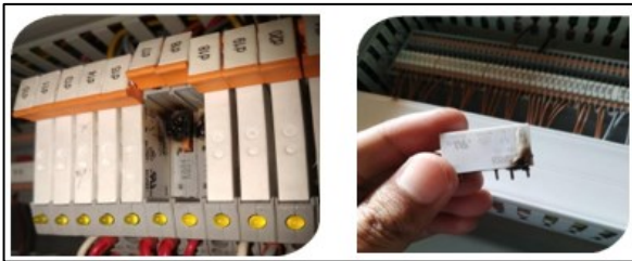
Gambar 7. Relay Aus/Terbakar
