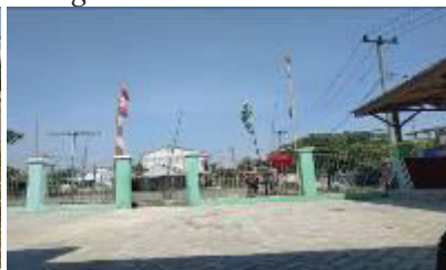
5. Proses pemasangan tower triangle .
